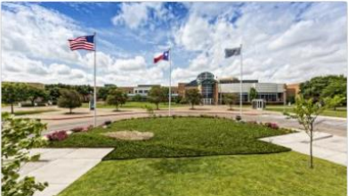
Southeast Campus: BAS Upgrades
