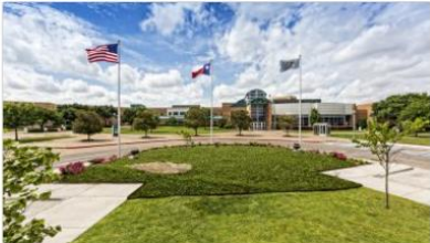
Southeast Campus: Emergency Power Upgrade - Generator
