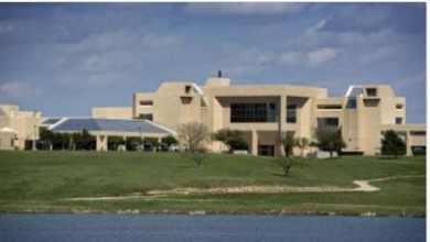
Northwest at Alliance: OWTL AHU/VAV Replacements - Phase I
