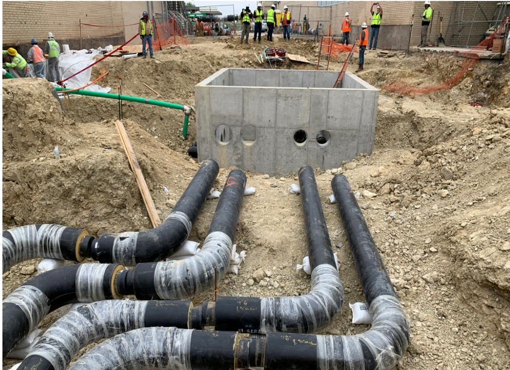
GMP 1: (Looking East) Summit Vault between WBSA and WCTS is installed and the thermal 4-pipe system installation in progress.
