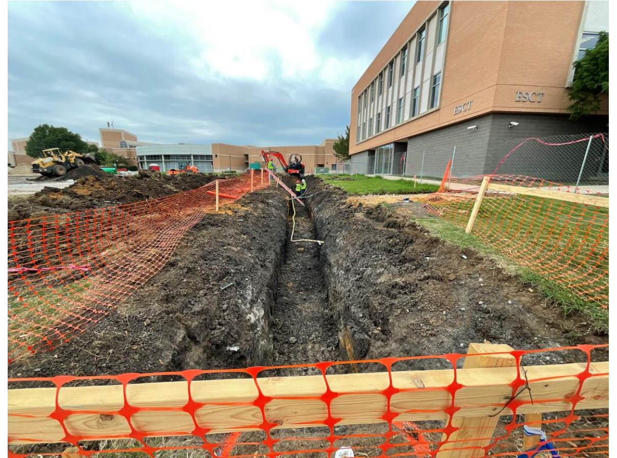
Gas line relocation in progress
